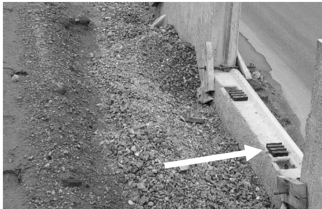
Fig. 5.4 Spacer strips placed between the panels
