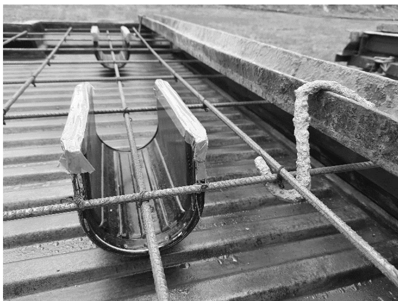
Fig. 2.8: SC Connectors with their openings sealed with tape
