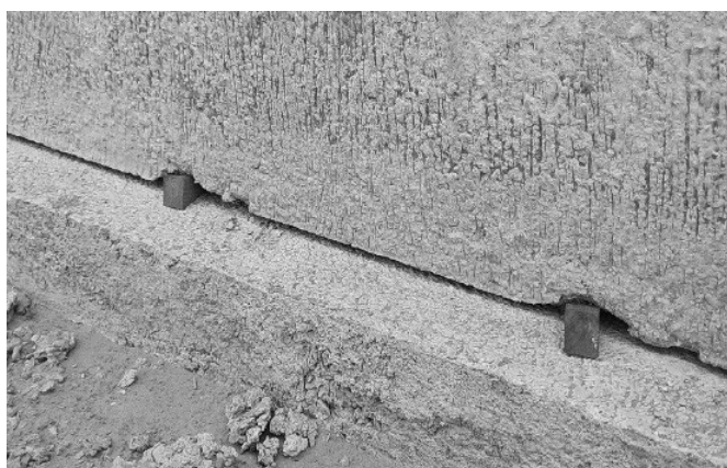
Fig. 5.5 Wooden wedges to hold panels in position
