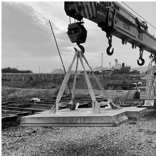
Fig. 3.13: Shifting of Panels for curing
