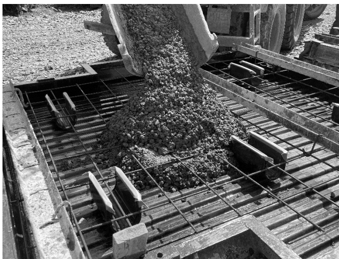
Fig 3.4: Concrete placement directly from Transit miller
