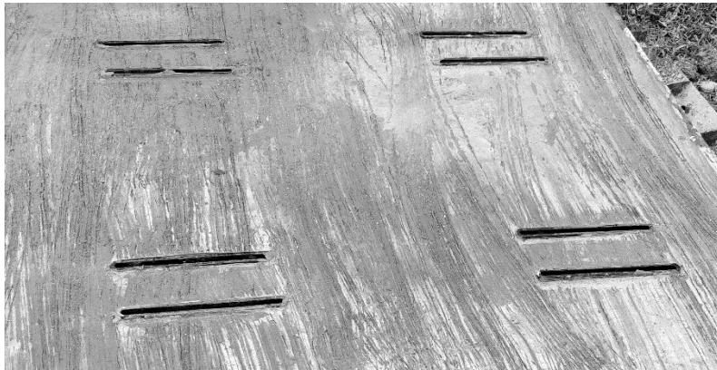
Fig. 3.9: After removing the tapes from SC Connectors
