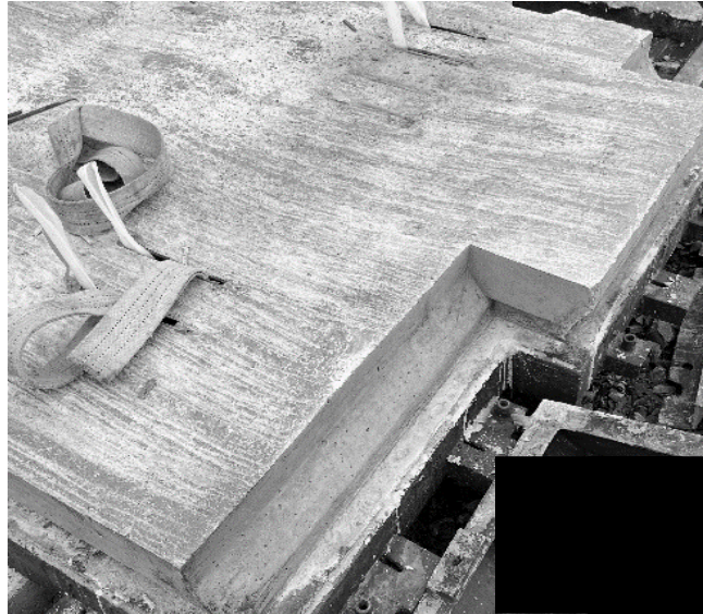
Fig. 3.11: Moulds Struck with care
