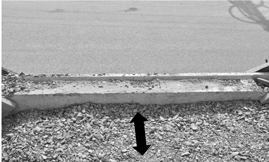
Fig. 2.9: Filter Medium adjacent to the Panel fascia
