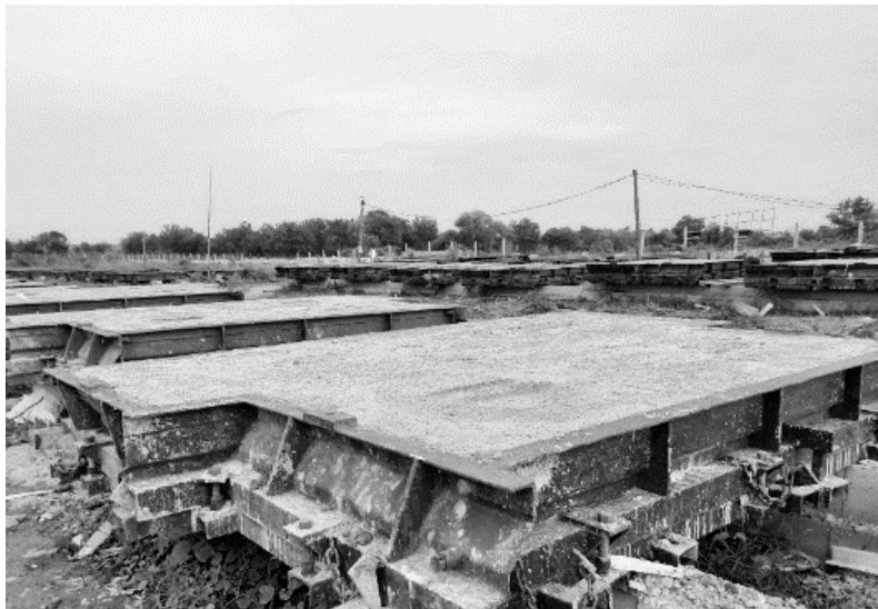
Fig. 3.10: Cast panels in moulds in casting line about 16 hours after casting and SC connector cavity covering tapes will be progressively removed
