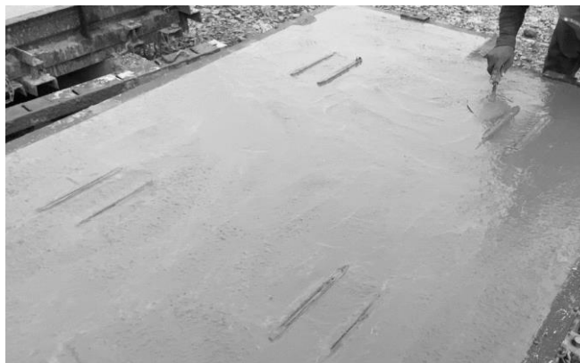
Fig 3.6: Concrete surface troweling
