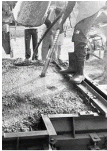
Fig 3.5: Concrete Compaction using a Needle Vibrator
