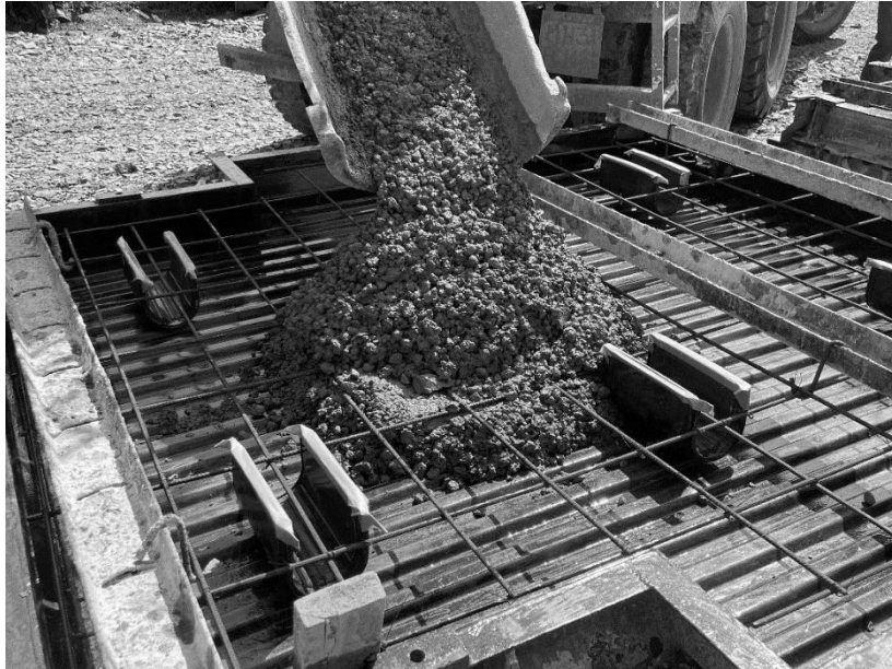
Fig. 3.8 : Concrete placement from a Transit Miller
