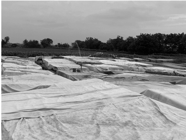
Fig. 3.14: Curing of Panels
