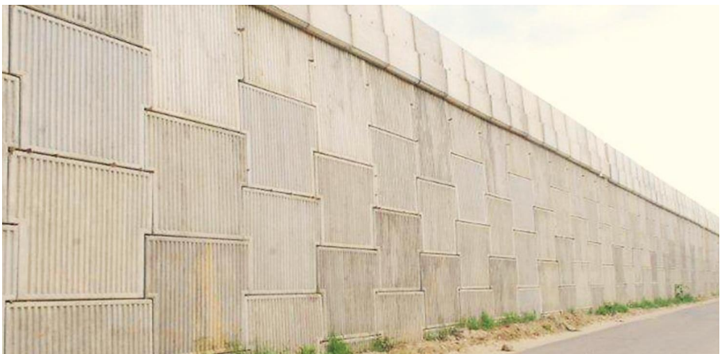
Fig. 5.14: The completed StrataWall™ EU system
