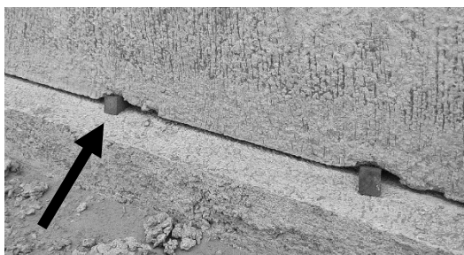
Fig. 2.10: Wooden wedges used for alignment
