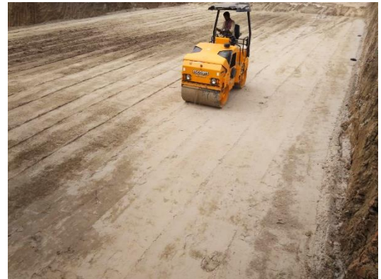
Figure 1 Preparation of subgrade
