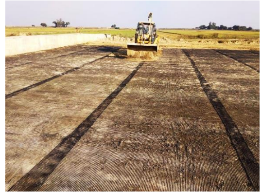
Figure 3 Filling of backfill material over StrataGrid™
