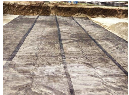
Figure 2 Laying of StrataGrid™ Biaxial Geogrid
