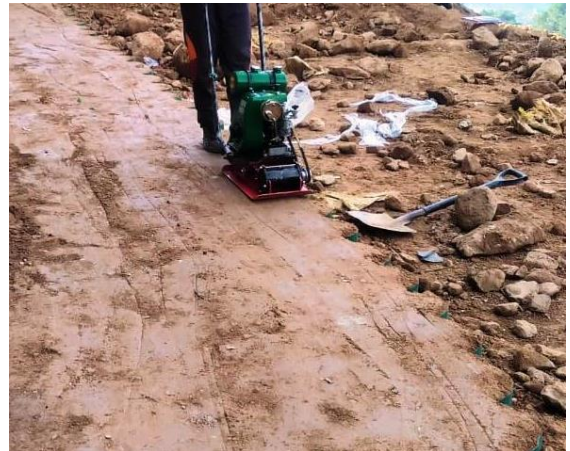
Figure 4: Compaction of infill material
