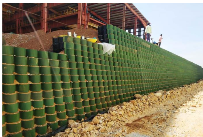
Figure 5: Gravity wall using StrataWeb® geocell
