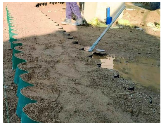
Figure 3: Infilling of StrataWeb® geocell
