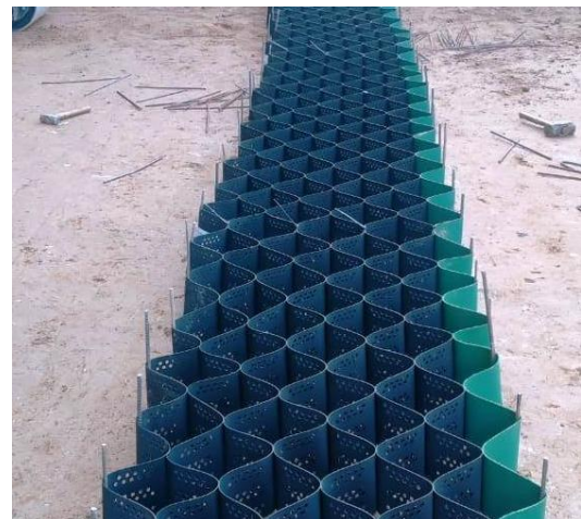
Figure 2: Installation of StrataWeb® Geocell Sections
